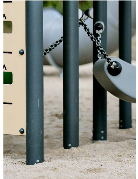
Hot-dip galvanised steel posts with powder coating to prevent corrosion.
